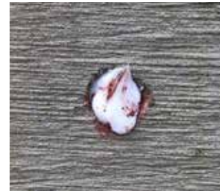
KÖSTER Crisin Cream is firm. This is an advantage when working from cartridges and tubular bags. Even when too much product is applied into the borehole, excess material will not run down onto the plaster that can lead to dark spots afterwards. Excess material can be removed and the borehole subsequently filled and plastered over.
