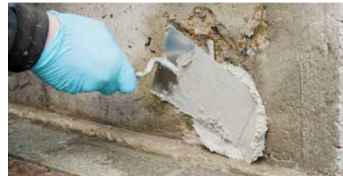
4 KÖSTER Betomor Multi A is applied with a spatula or a trowel in one step.
