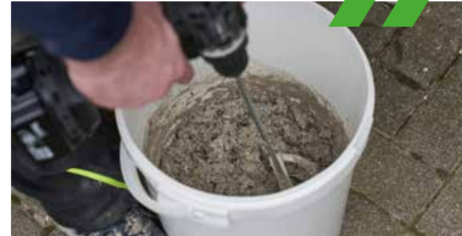
2 Mix KÖSTER Betomor Multi A with clean water (4.5 l per 25 kg bag; 2.7 l per 15 kg bucket) to a smooth, lump-free mass.
