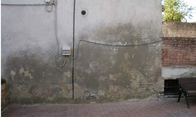
Change of color, reduction of the thermal insulation
