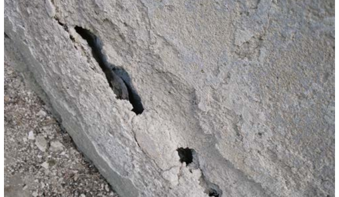
Damaged plaster
